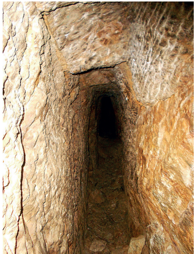
Fig. 22. Manually excavated medieval mining galleries “kresanica” with a hammer and pick technology in the underground of Ľubietová (Podlipa), photo P. Hronček
